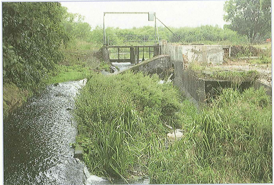
Dams at old mills have prevented fish migration. According to the Gudenaa Committee recommendation, most of these fish passage obstacles have been removed.
