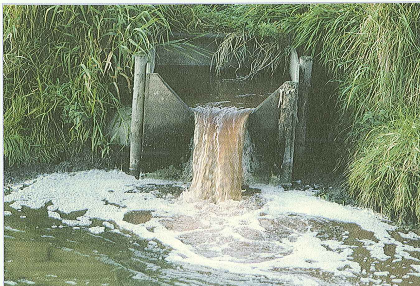
Wastewater discharge from a slaughterhouse to Lilleaa 1976. Photo: Bent Lauge Madsen
